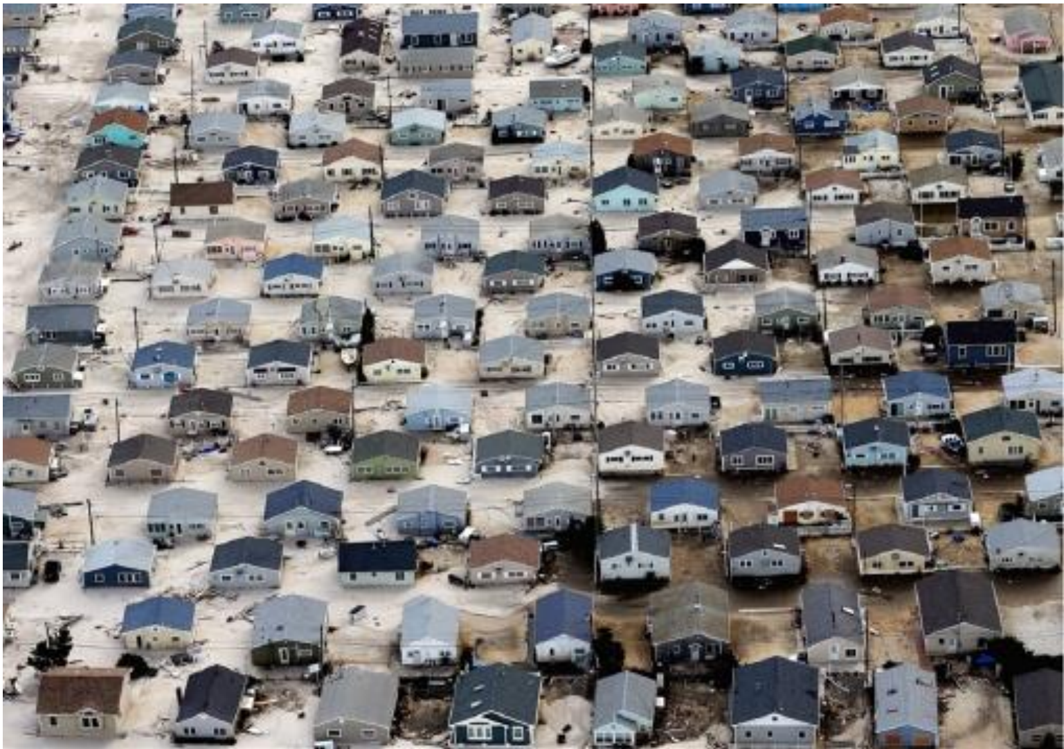
New Jersey overwash from Super Storm Sandy
