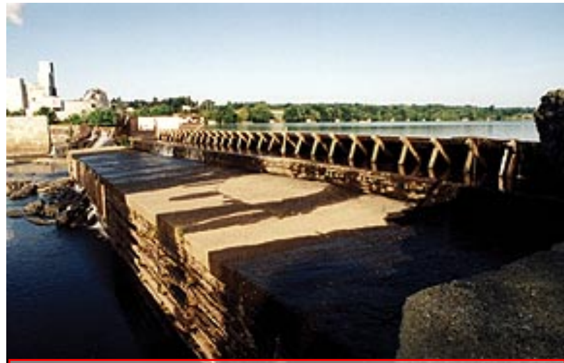
Greatworks Dam, Penobscot River
